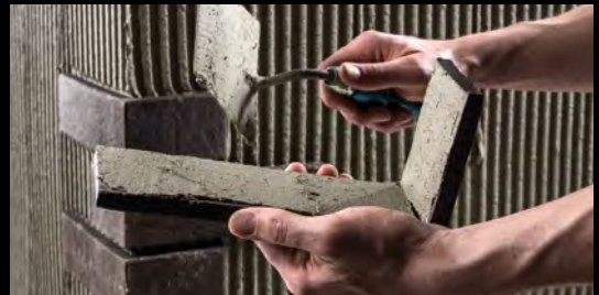
The corner angles are worked using the floating-buttering method.
