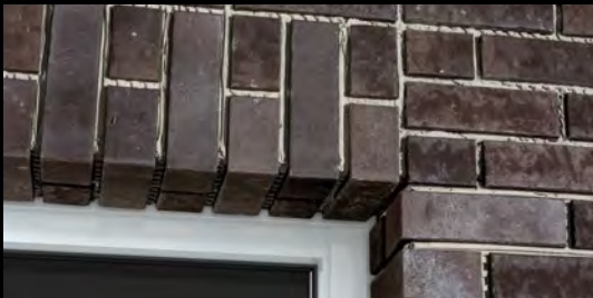
Window lintel perfectly replicated with angles.
